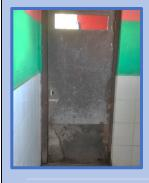
The bathroom is in urgent need of repair work, including replacing the toilet seat, toilet, bathroom door, and taps. The current fixtures are damaged and affecting the functionality and aesthetics of the space. It is crucial to install new aluminum doors that are water-resistant to prevent further damage. However, due to budget constraints, the necessary repairs cannot be completed at this time, despite the urgency of the situation.
